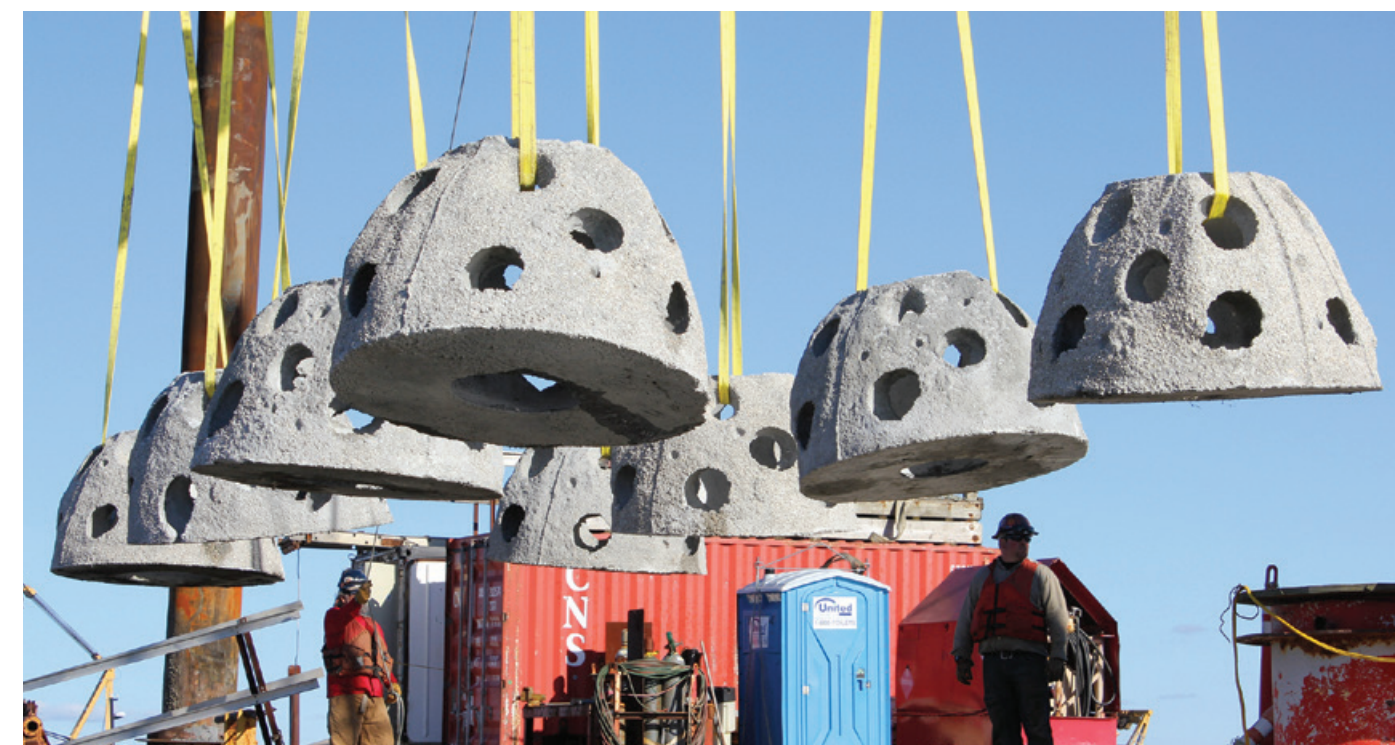
Placing reef balls at Sabin Point in Riverside, Rhode Island. © Timothy Mooney/TNC
